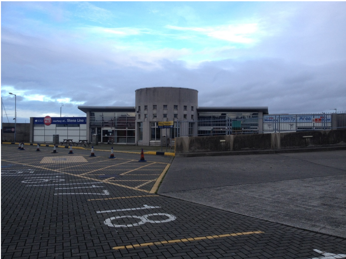
Figure 10.5.2 – Modern building within the development area, facing north
