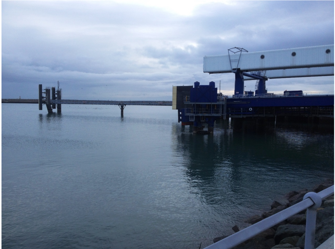
Figure 10.5.4 – Existing berth and walk way, facing ENE
